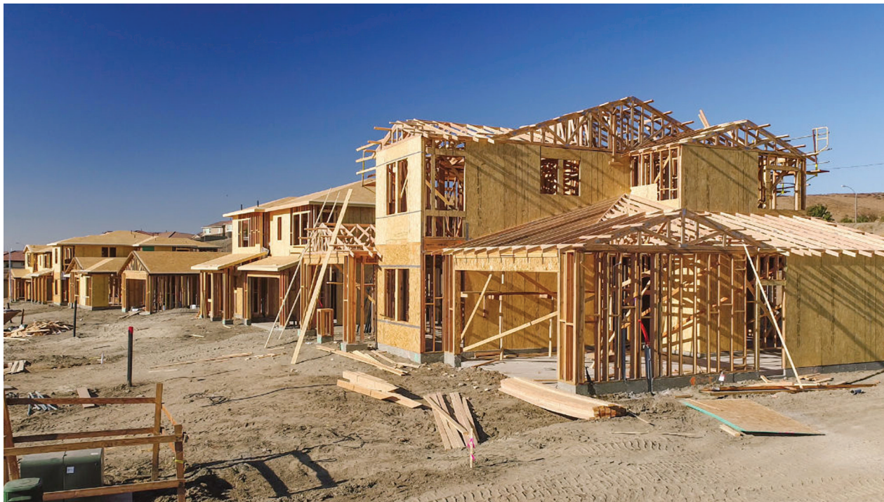
New residential construction near Oklahoma City.
